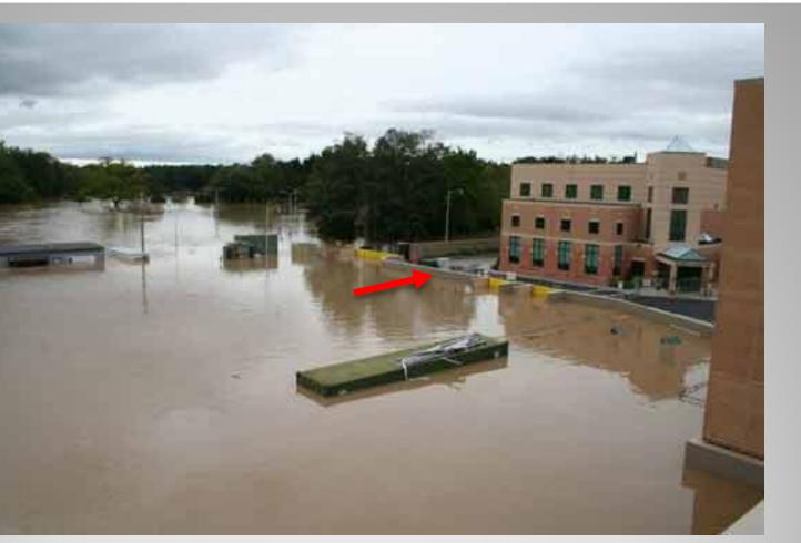
Water from Susquehanna River flooding rear parking lot. Flood wall proves to be very effective.
